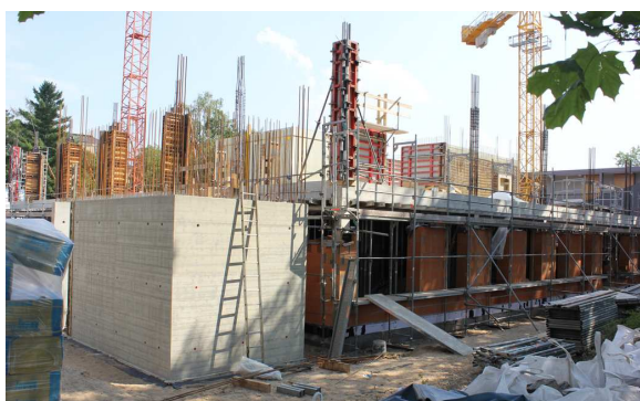
CSBD building construction, August 14, 2015. Picture by K. Boes, MPI-CBG.
